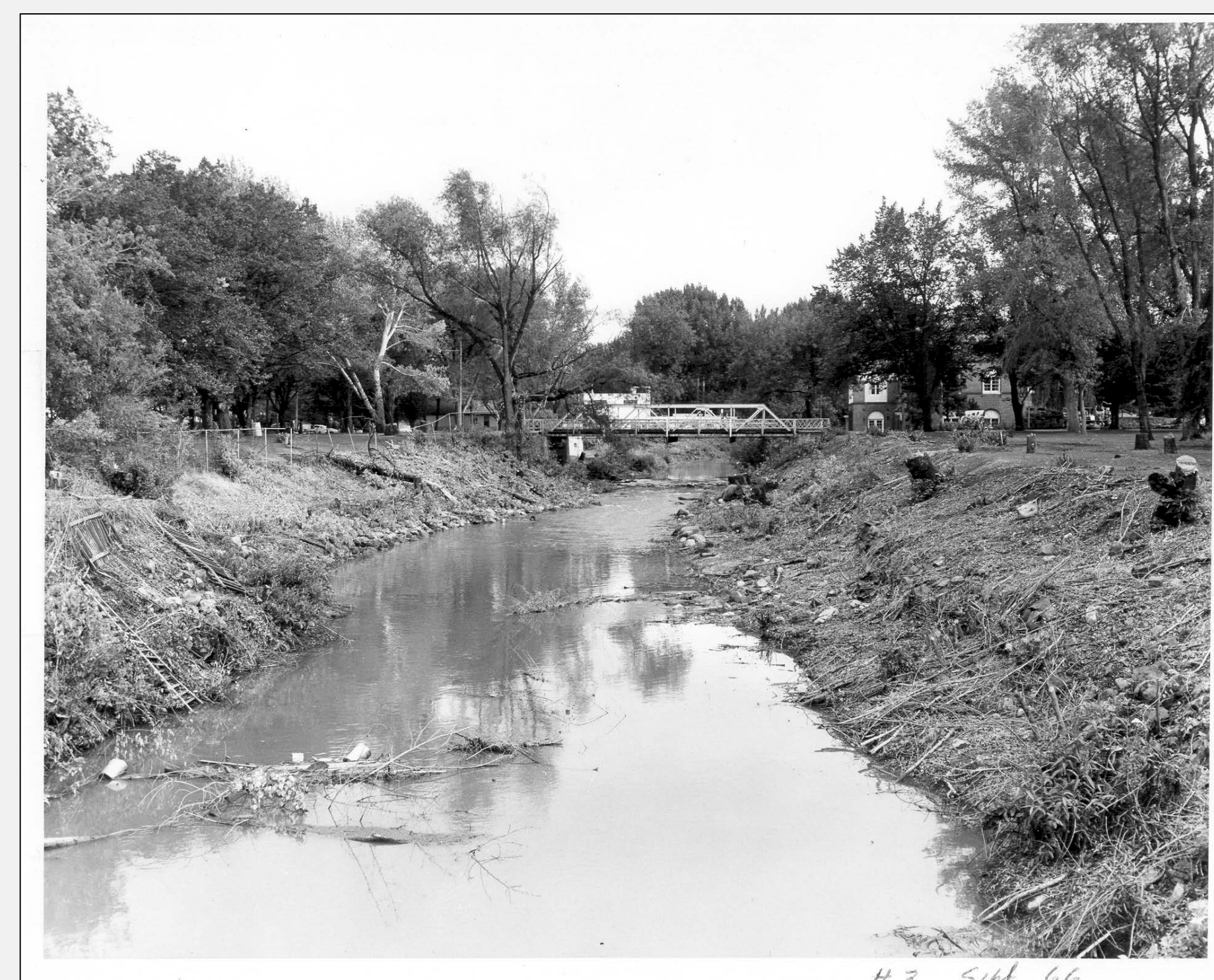
Figure 3. A 1966 photograph looking towards Freemont Street and the Veteran's Memorial Building in Pocatello, Idaho. Note the channel under construction with tree stumps lining the edges of the riverbed. Source: U.S. Army Corps of Engineers. “Portneuf Basics” of Portneuf Visioning Study website.
